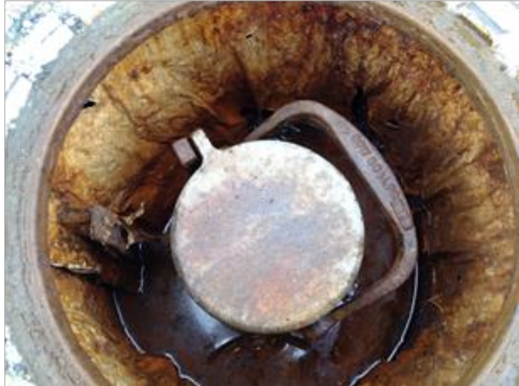
Figure 4: Picture of a Corroded Spill Bucket UST Found in April 2016 For Which Follow-Up to Determine if the Violation was Corrected Was Not Performed
